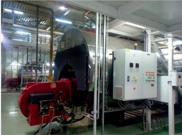
**Fig. 6:** 5 MW dual-fuel burner converted for CO<sub>e</sub>/O<sub>2</sub> optimisation with LT3F sensor electronics and switch cabinet with integrated BT300, speed control, etc.
