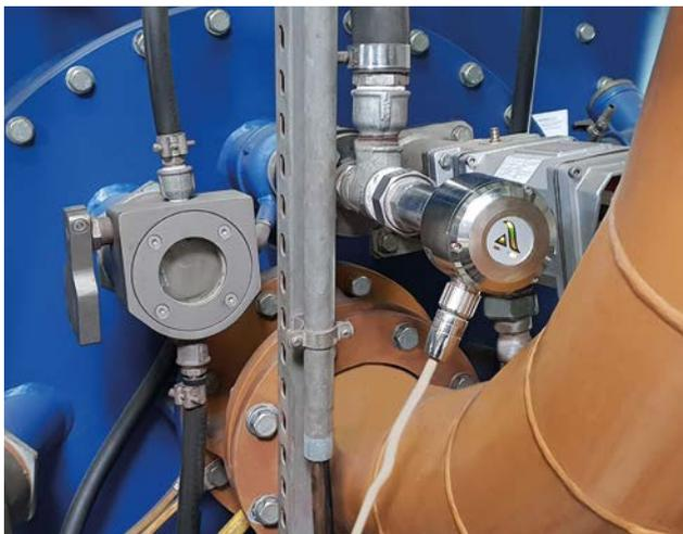
The LAMTEC F200K flame scanner in operation.
