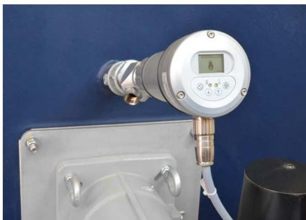
The LAMTEC F300K flame scanner in operation.
