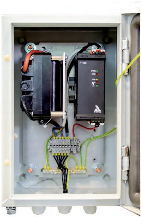
Fig. 3-32 External power unit safe area
