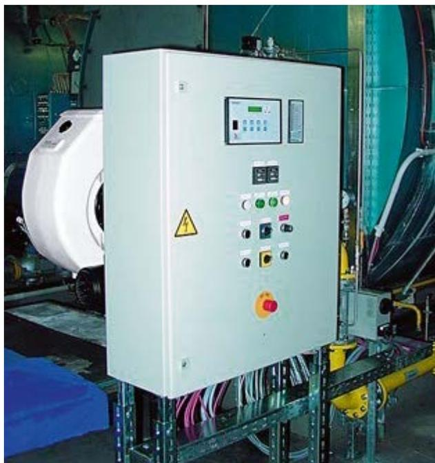
entire control directly on the burner and still take advantage of bus networking and PC-based remote control, evaluation and documentation via defined interfaces.
